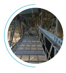
The system replaces traditional suspended scaffolding for under deck working areas on bridges, jetties and ports, providing a safe working platform, designed to suit almost any shape of size of application.
