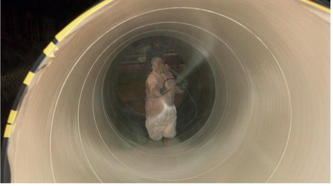
Humidur FP Quick Repair (QR), has been applied on the pipe work of Shell's Mossmorran plant.
