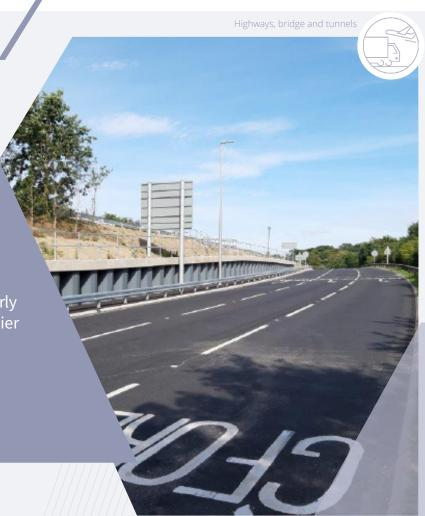
The primary works included widening the existing slip road and undertaking a number of upgrades to bring the road, in line with current national design standards. Works began by the team upgrading the existing drainage system from a gulley system to a combined kerb and drainage system, with necessary upgrades to the existing vehicle restraint system.
