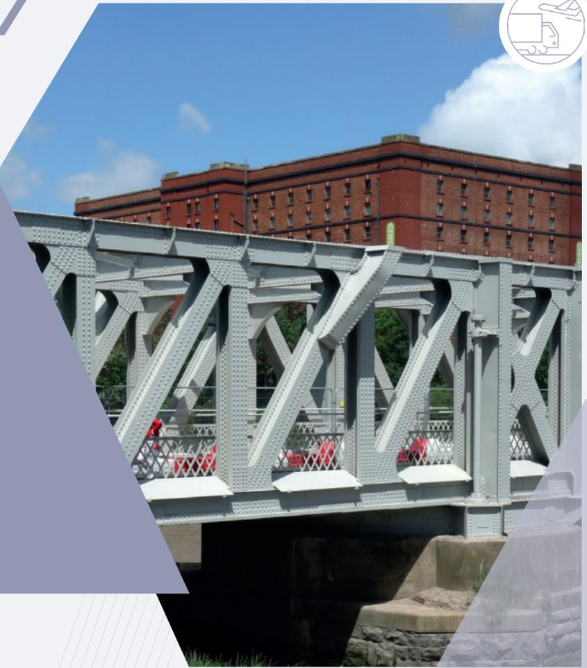
Built in 1906, this former road and rail swing bridge over the River Avon in Bristol, formed part of a local access and cycle route, despite being in a poor state of repair. The Grade 2 listed bridge was on Bristol City Council's 'Listed Building At Risk Register', which described the bridge as being in a very bad condition with clear signs of structural instability. The register stated that, prior to works taking place, the bridge was at "immediate risk of further rapid deterioration".
