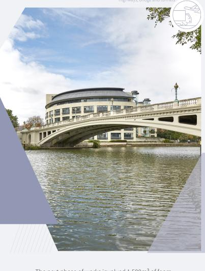
The next phase of works involved 1,500m³ of foam concrete being pumped into the south approach ramp and cored through the deck before it was filled in from the top. Following a three-month waiting period, to allow the concrete to settle, the team then applied a grouting product, as well as using a sheer bolt system to thicken the abutments, strengthening the entire structure.
